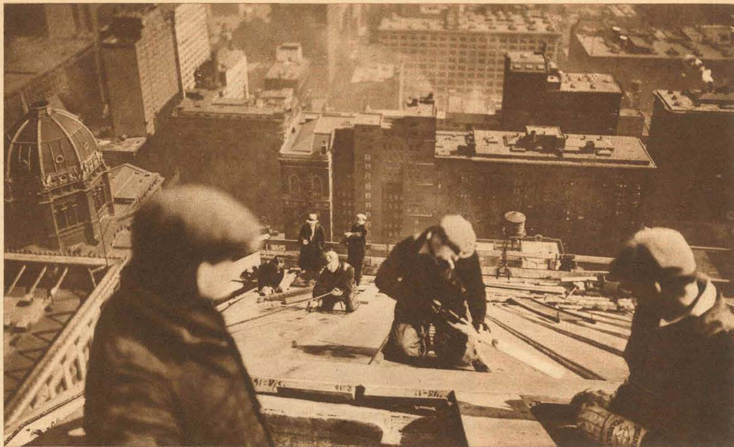
Dachreparaturen in 150 m Höhe
